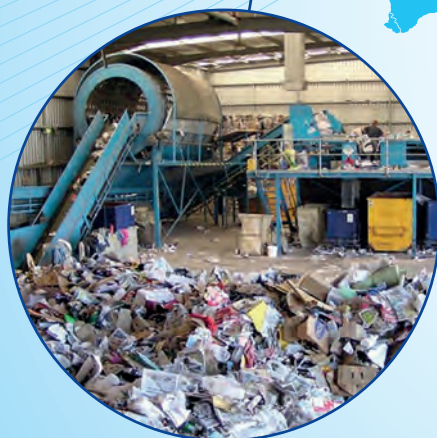
Waste processing plant 垃圾处理厂
