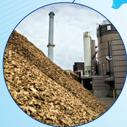
Biomass Power Station 火电站
