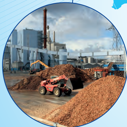
Biomass Power Station 火电站
